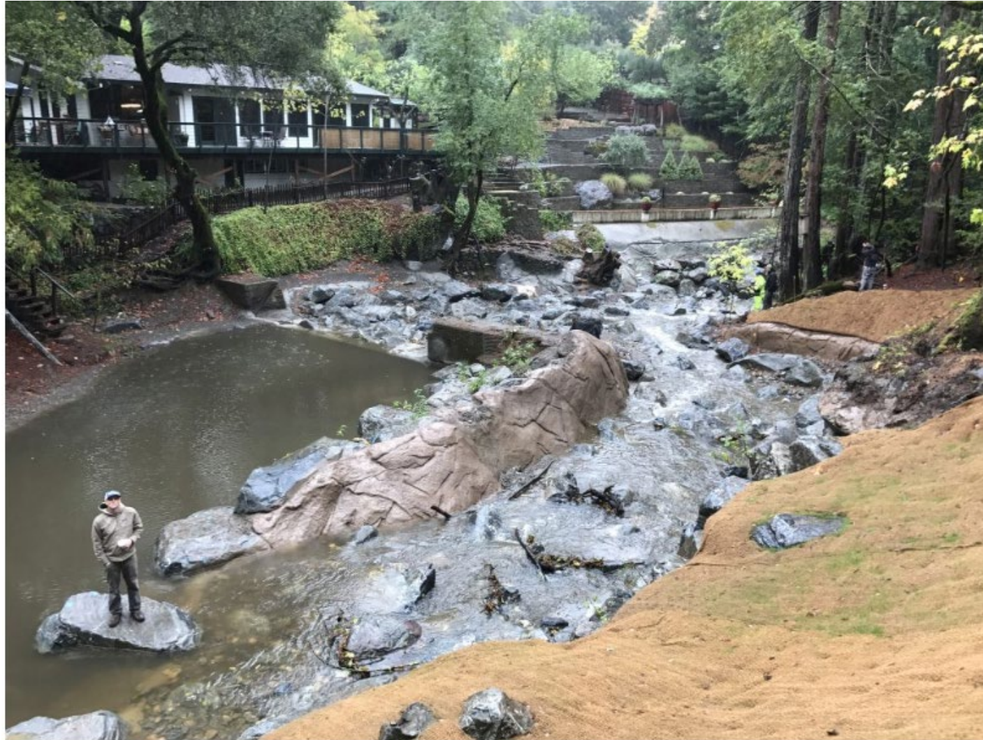
The site after construction.
